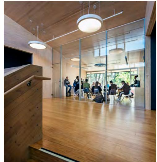
Black spruce CLT panels act as the tension surface (and final ceiling finish) in a system of prefabricated stressed skin assemblies that span the upper classrooms and circulation spaces. Vertical CLT panels form bearing and shear walls throughout the building.
