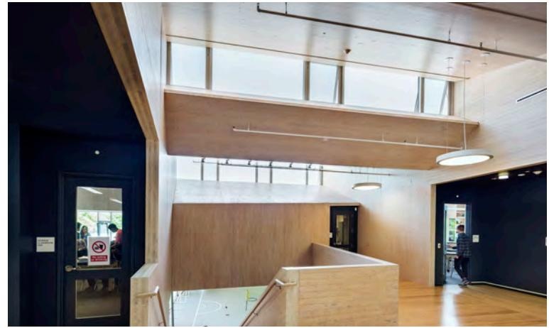
The sawtooth roof provides diffuse natural lighting for key spaces, allows for simple installation of photovoltaic panels on the south facing slopes, and directing water to the surrounding rain gardens. The architect says artificial light is sparingly used, helping reduce energy expense and improving student and faculty visual comfort.
