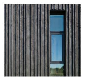
The salvaged timber was milled to board and batten siding, then charred and sealed using a traditional Japanese burning technique, shou sugi ban. The burn adds a layer of carbon which removes water from the wood. The carbon also protects against mold, rot, and insects, as well as fire.
