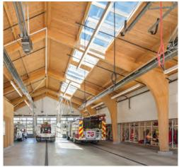
The glulam arches serve as part of the primary structural frame and were designed to resist vertical and lateral loads, with additional structural factors of safety required for Essential Facilities under the Oregon Structural Specialty Code (Building Code).
