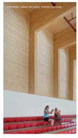
The Martha C. Cutts Gymnasium is a one-story structure with a roof that slopes from 32 feet to 27 feet. There are 12 structural bays, including the ends, with 75-foot long glulam beams. The beams are a single continuous piece. There are 36 glulam columns. CLT is used for both wall and roof panels. All CLT is 3-ply with slightly varying thicknesses.
