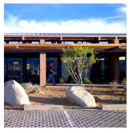
Extended wooden trellises form a shaded outside perimeter, helping manage solar gain and limiting interior cooling and lighting expenses.
