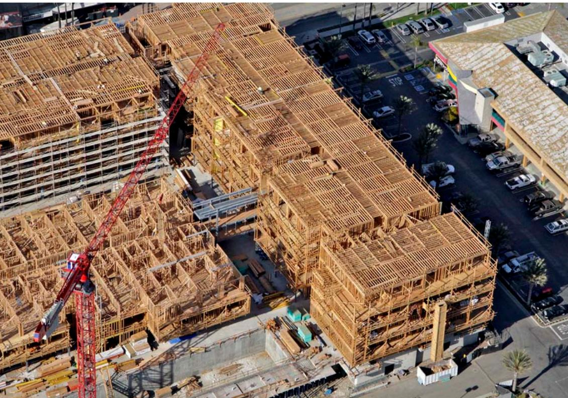
Finn said they were deliberate in their decision to use the right building component in the right application. "Each wood component had its place in Stella. Most of the floor assemblies were 11-7/8-inch I-joists; we used exposed glulam beams in the public spaces, and we used LVL where we had higher load concentrations. We specified fire-retardant-treated (FRT) wood components for the exterior walls of the Type III-A structure, and non-treated dimension wood everywhere else."
