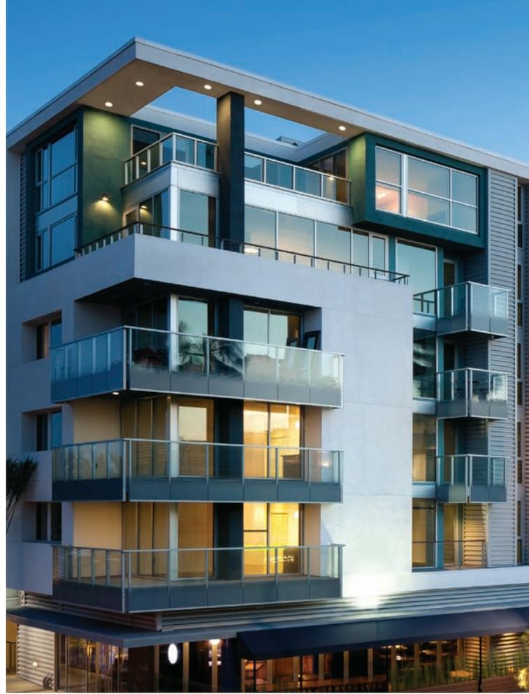
timber (Type IV) construction, or if automatic sprinklers are used, the balcony may not need to be protected. To avoid fire rating requirements, Stella’s balconies were protected with automatic sprinklers.
