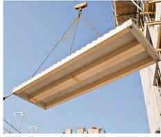
Hybrid floor slab features wood-concrete composite rib construction. Photo Credit: www.creebuildings.com
