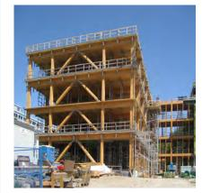
Exposed view of glulam chevron braces at UBC Earth Sciences Building Architecture by: Perkins+Will Photo credit: Equilibrium
