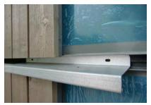
Holz8 exterior wood façade with metal flashing between each storey prevents the spread of fire Photo credit: Huber & Sohn
