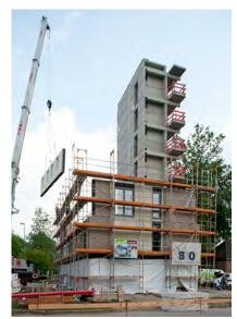
Prefabricated panel installation at Holz 8 Architecture by: Schankula Architekten Photo credit: Huber & Sohn
