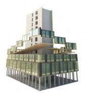
Modular system of interlocking prefabricated components with centralized concrete access core. Detail Credit: www.creebuildings.com
