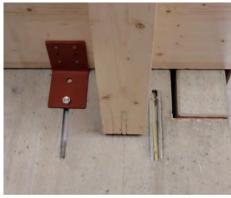
Steel bracket used to connect wood floor panels to concrete core. Photo credit: Huber&Sohn
