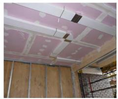
Building systems are routed through a ceiling void created with gypsum board. Photo credit: Willmott Dixon Group
