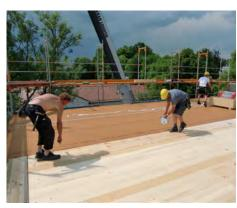
Floor panels covered with waterproof membrane after installation. Photo credit: Huber&Sohn
