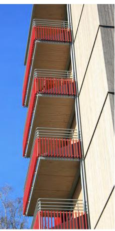
Timber balcony panels enclosed by steel frame Photo credit: naturally: wood
