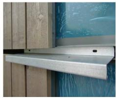
Metal flashing between each storey prevents the spread of fire. Photo credit: Huber&Sohn
