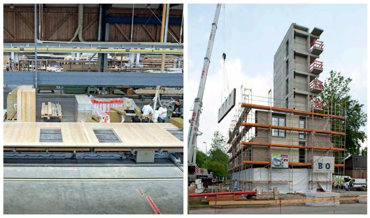
Left: Prefabrication of wall panels. Right: Timber erection time took 2 days per level. Photo credit: Huber&Sohn
