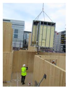
Installation of prefabricated bathroom pod at Forté. Photo credit: Lend Lease
