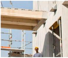
Angled steel brackets connect hybrid floor slabs to concrete access core. Photo Credit: www.creebuildings.com
