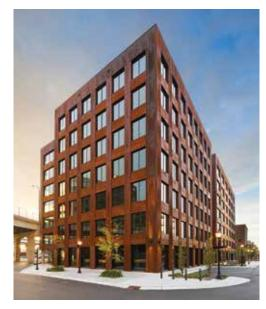
Approximately 3,600 cubic meters of wood are used in the T3 office building, in Minneapolis, which will sequester about 3,200 tons of carbon for the life of the building. The seven-story, 220,000-square-foot commercial building offers a mix of retail and office space.
