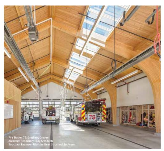
Part of the structural system, the arches in this apparatus bay are designed to resist vertical and lateral loads required for essential facilities under the Oregon Structural Specialty Code. This project won a 2016 WoodWorks Wood Design Award. Photo credit: Josh Partee Photography
