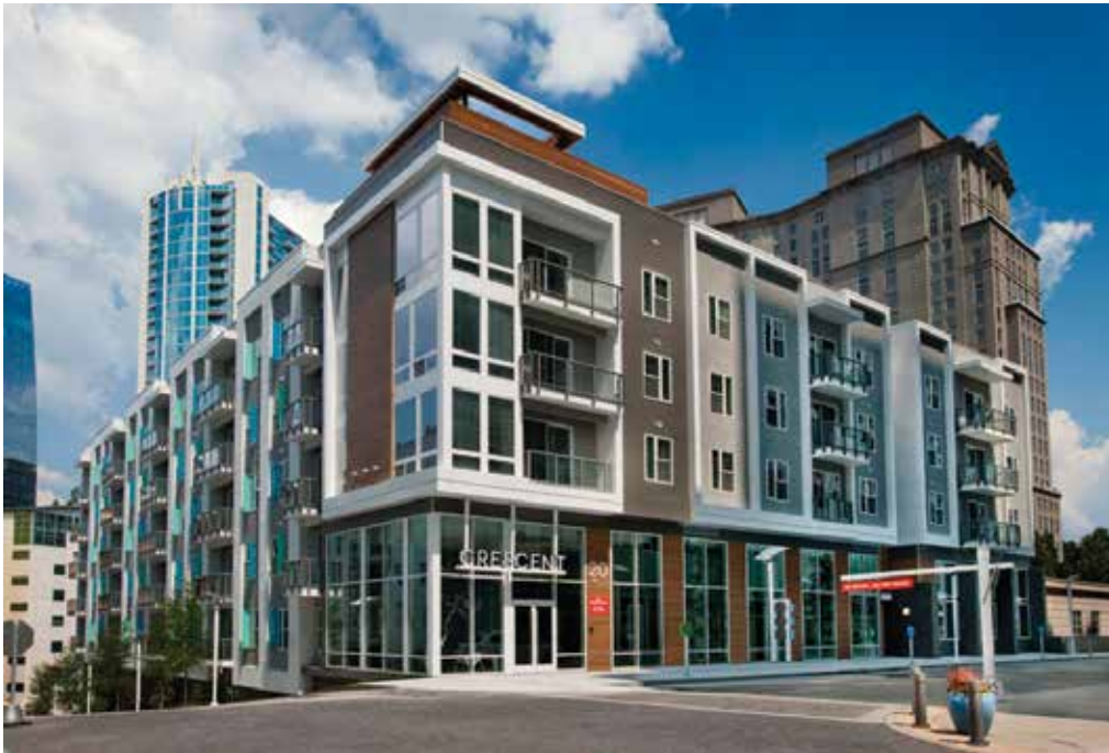
Carbon Benefits: Crescent Terminus – Atlanta, Georgia; Architect: Lord Aeck Sargent. According to the Wood Carbon Calculator for Buildings ( www.woodworks.org ), Crescent Terminus has a carbon benefit equivalent to 2,583 cars off the road for a year or the energy to operate a home for 1,149 years. Photo by Richard Lubrant
