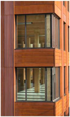
T3 is made chiefly with nail-laminated timber (NLT). Over 1,100 8-foot wide by up to 40-foot long NLT panels were used for exposed structural ceiling and roof panels with concrete topping. Spruce was used for the glulam beams and columns. "The texture of the exposed NLT is beautiful," notes Candice Nichol, project lead and architect for MGA. "The small imperfections in the lumber and slight color variation adds to the warmth and character of the space."
