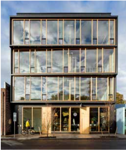
Left exposed, visible wood structural elements offer impressive visuals that accentuate a project's design and improve occupant health and well-being. Albina Yard | Lever Architecture. Photo courtesy of LEVER Architecture
