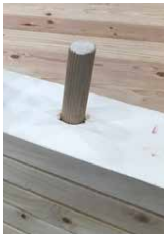
DLT is similar to NLT but instead of nails or screws, DLT uses wood dowels to join laminations. Photo courtesy of Think Wood
