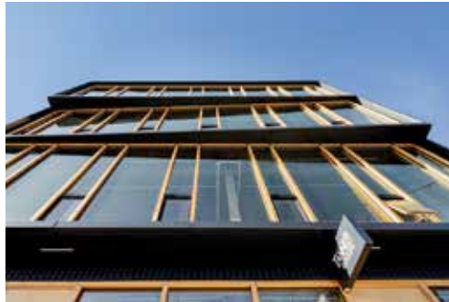
The relative lightness of CLT panels and beams permitted a smaller foundation, which can preclude the need for expensive piles or allow a taller structure. Albina Yard | Architect: LEVER Architecture | Photo: Jeremy Bitterman, courtesy of LEVER Architecture
