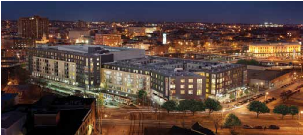
The Fitzgerald capitalizes on the benefits of podium design to create sustainable mixed-use living. The podium maximizes versatility, transferring loads from four wood stories above to a 30-foot grid to achieve higher densities and allow a mix of commercial, residential and parking. The Fitzgerald | Architect: Design Collective | Photo: Richard Greenhouse
