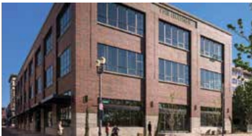
Because of its strength and dimensional stability, mass timber offers a low-carbon alternative to steel, concrete and masonry for many applications. The Hudson | Architect: Mackenzie Architects | Photo: Christian Columbres Photography
