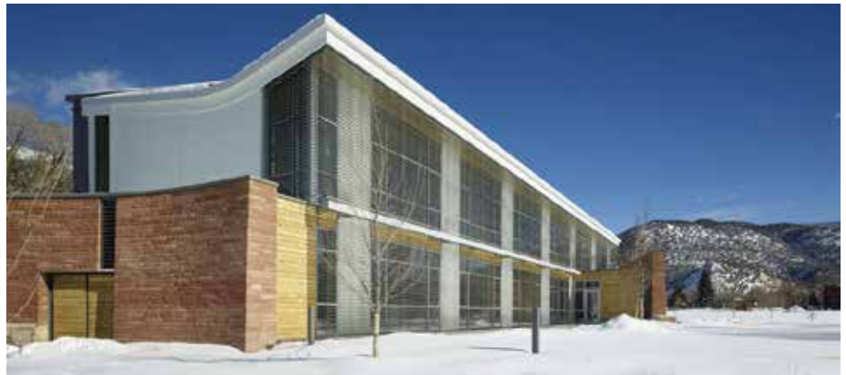
Wood is a strategy used to denote building entries and as a transition between exterior materials.
