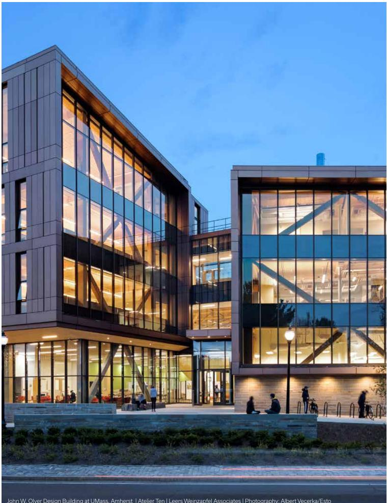
The 87,000 square foot facility is one of the **most advanced CLT buildings** in the U.S. and saves the equivalent of **over 2,300 metric tons of carbon** when compared to a traditional energy-intensive steel and concrete building.
