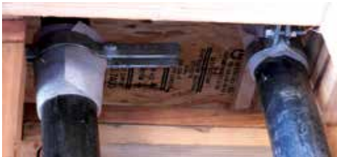
Plumbing sleeve connected to structure with foam wrap to allow for vertical movement of structure
