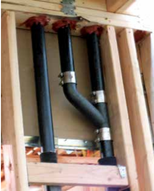
Plumbing joints with pipes nested in joint to allow for vertical movement of structure
