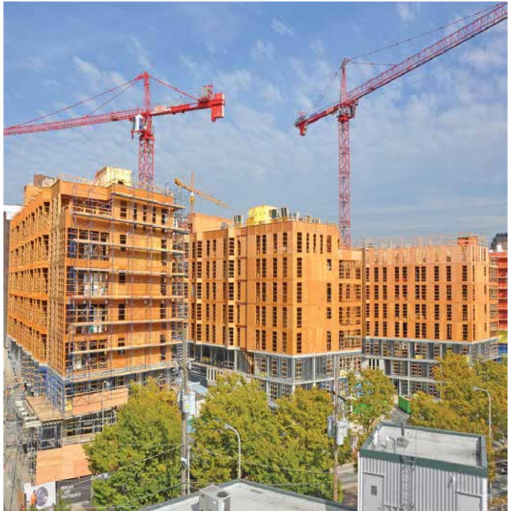
Mercer Court at the University of Washington includes five buildings, each with five stories of wood-frame construction over two or three stories of concrete. Photo: W.G. Clark Construction, Ankrom Moisan Architects
