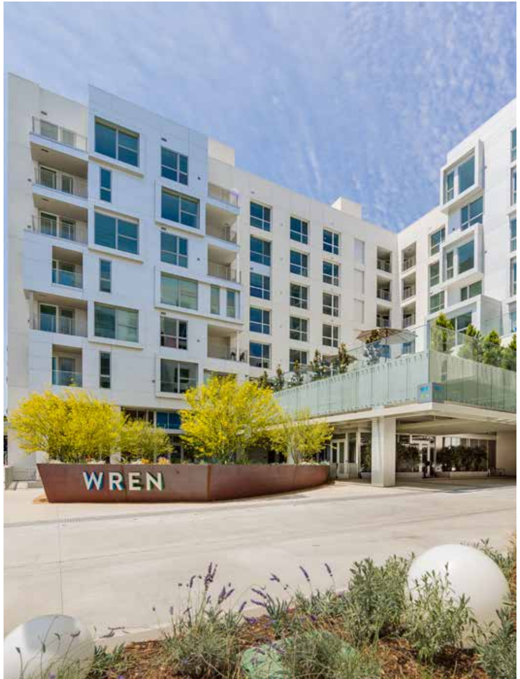
The wood-frame, residential building, WREN, located in Los Angeles, CA, is one of the first of a new building type using multiple podiums. By providing a sprinkler system, a type III construction, and multiple building modifications, the wood portion of the building was able to increase from 4 stories to 5 stories. Architect: Togawa Smith Martin Inc. Photo: Kevin C. Korczyk
