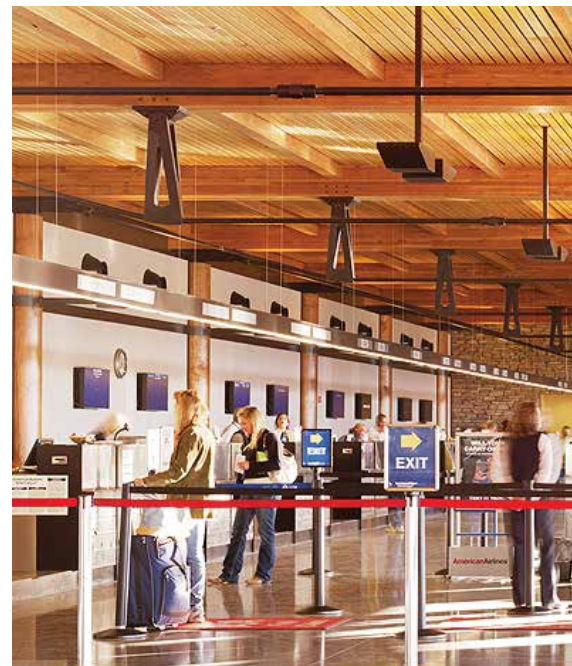
ABOVE: For the Jackson Hole Airport in Wyoming, designers chose wood because of its varied grain and color palette, as well as its ability to perform structurally under a variety of loading conditions. The inherent fire performance of heavy timber construction was vital in allowing the wood to be exposed. Winner of a 2015 WoodWorks Wood Design Award.
