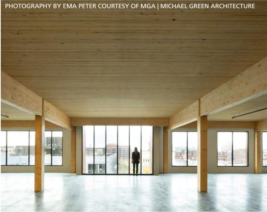
Exposed NLT panels, beams, and columns meet all aspects of code, including fire. Mass timber has different burn characteristics than light-frame lumber and building and fire code recognizes that tested life safety margin. Charring is the difference. A charred timber retains most of its mass and strength at a predictable rate, with surface charring acting as a fire insulating material.
