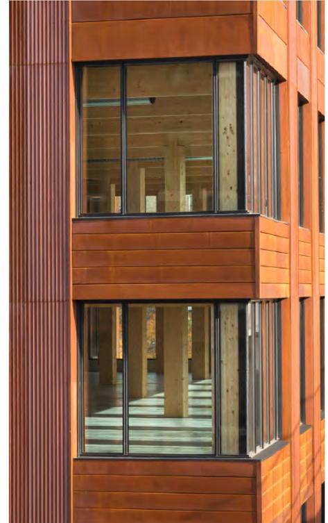
T3 is made chiefly with nail-laminated timber (NLT). Over 1,100 8-foot wide by up to 40-foot long NLT panels were used for exposed structural ceiling and roof panels with concrete topping. Spruce was used for the glulam beams and columns. "The texture of the exposed NLT is beautiful," notes Candice Nichol, project lead and architect for MGA. "The small imperfections in the lumber and slight color variation adds to the warmth and character of the space."
