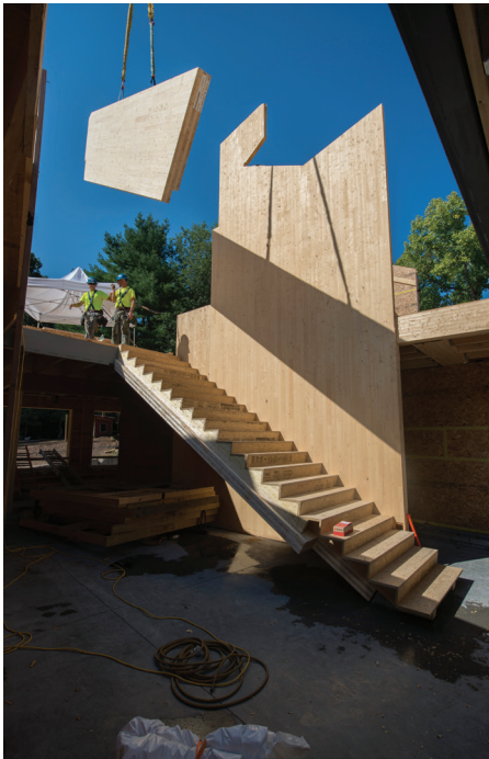
A new addition to Common Ground High School in New Haven, Conn., was framed using heavy timber and mass timber components in just four weeks.
