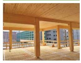
Designed by MGA, the seven-story T3 building in Minneapolis, Minnesota, includes glulam columns and beams, and NLT floors. Photo courtesy of StructureCraft
