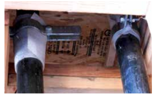
Plumbing sleeve connected to structure with foam wrap to allow vertical movement of structure
