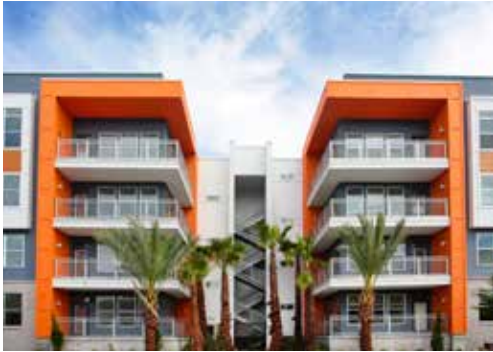
2016 Wood Design Award Winner: Brooklyn Riverside, Jacksonville, Florida. Architect: Dwell Design Studio. Photo: Pollack Shores, Matrix Residential
