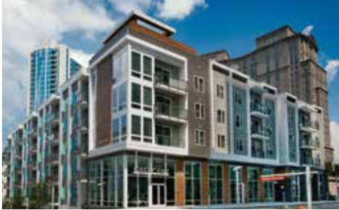
Berkshire Terminus, Atlanta, Georgia. Architect: Lord Aeck Photo: Richard Lubrant
