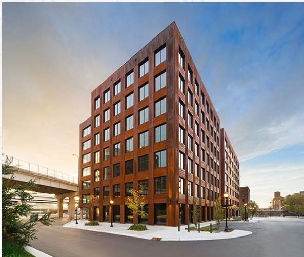
T3 | Photography Courtesy of Ema Peter and Wood Specialist Consultant Architecture firm MGA | Michael Green Architecture
